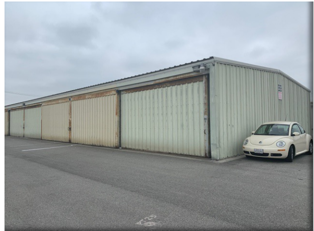
Permanent T-Hangar (Large) Row BB
