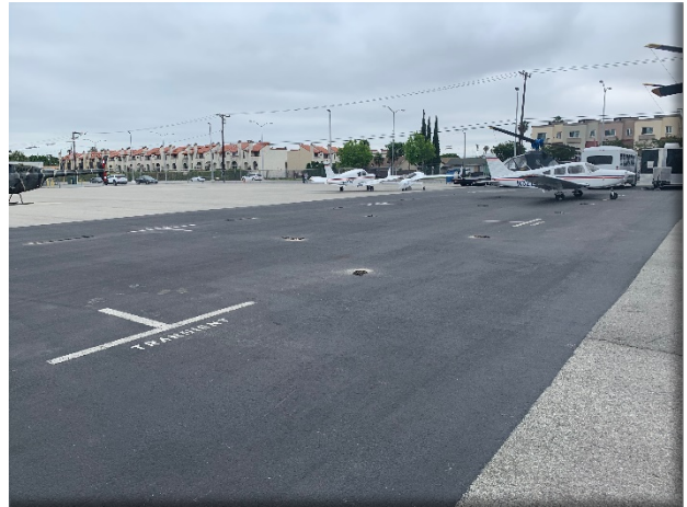
South Tiedown area
